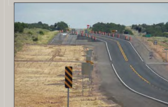
Reconstruction of US 82 will be completed in two phases.
