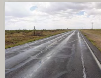
Roadway conditions east of Maljamar.
