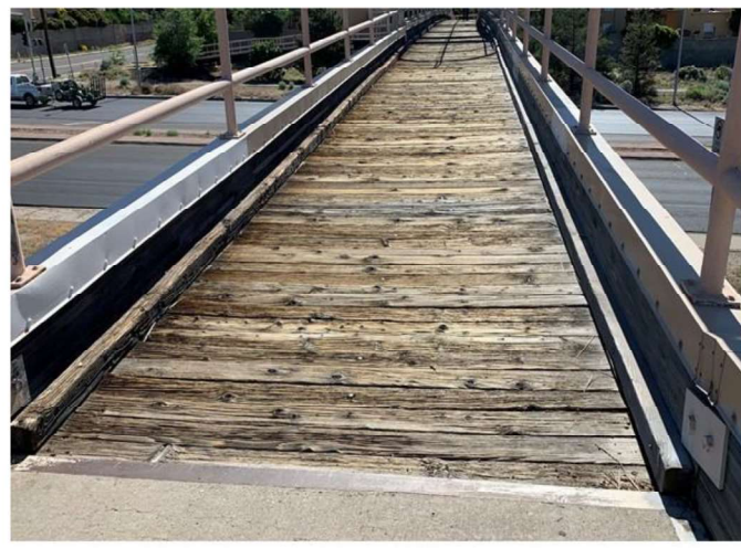
Existing timber bridge decking
