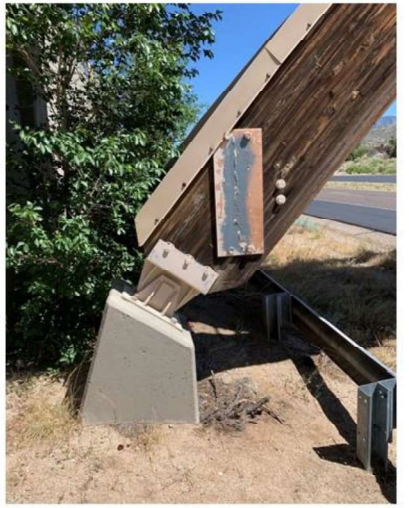
Existing steel bridge elements
