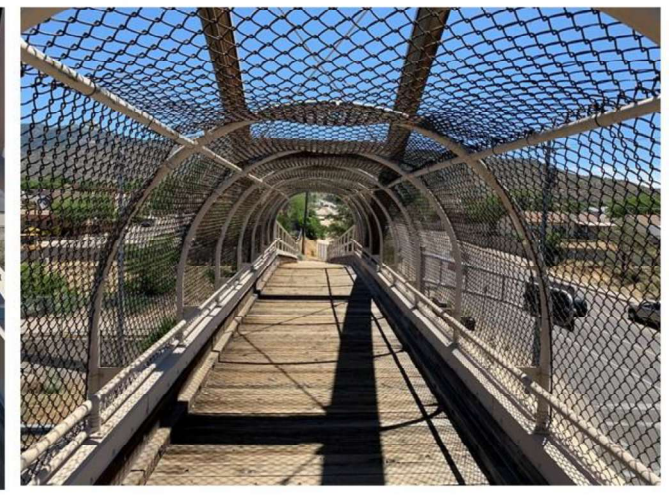
Existing pedestrian fence
