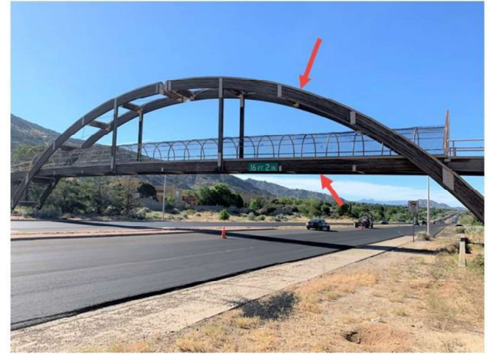
Existing timber glulam beams
