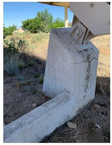
Existing concrete bridge elements
